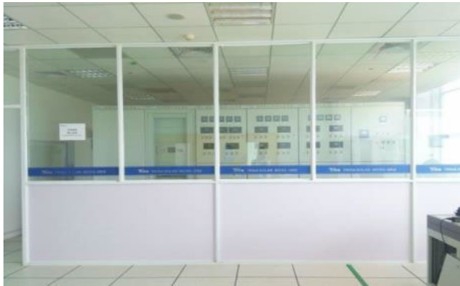
Capacity : 30 kW / 100 kWh Type: PV + Storage + Diesel
