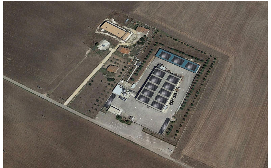
Italy «industrial factory» Location: Bari, Italy Project Type: Roof Top Project Scale: 499,2 kWp
